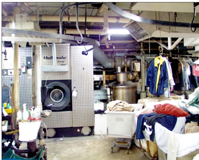
Dry cleaning operation
